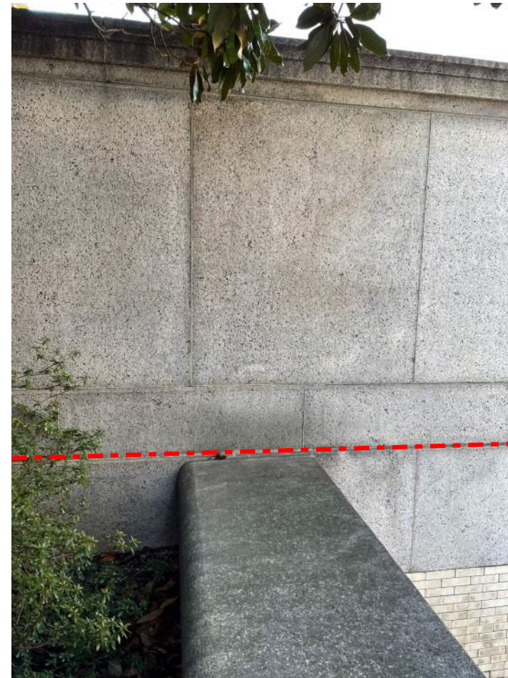
VIEW D (looking Northwest)
