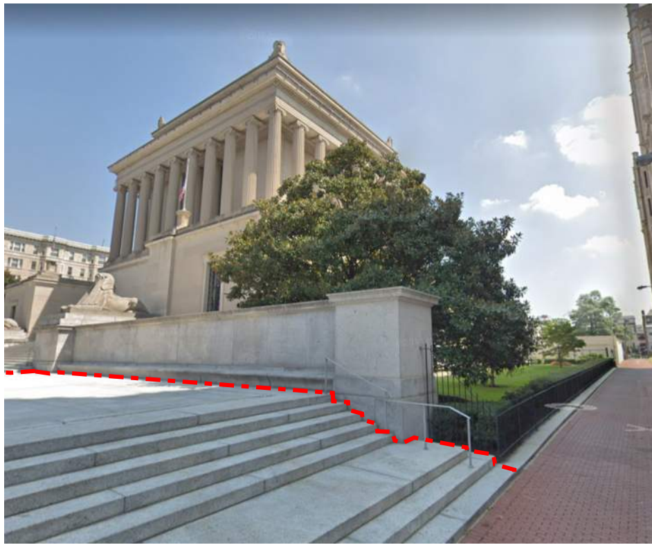
VIEW A (looking Northeast)
